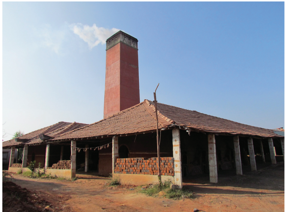
The search for a cleaner brick production regime is a key to reducing emissions and saving precious coal and clay
